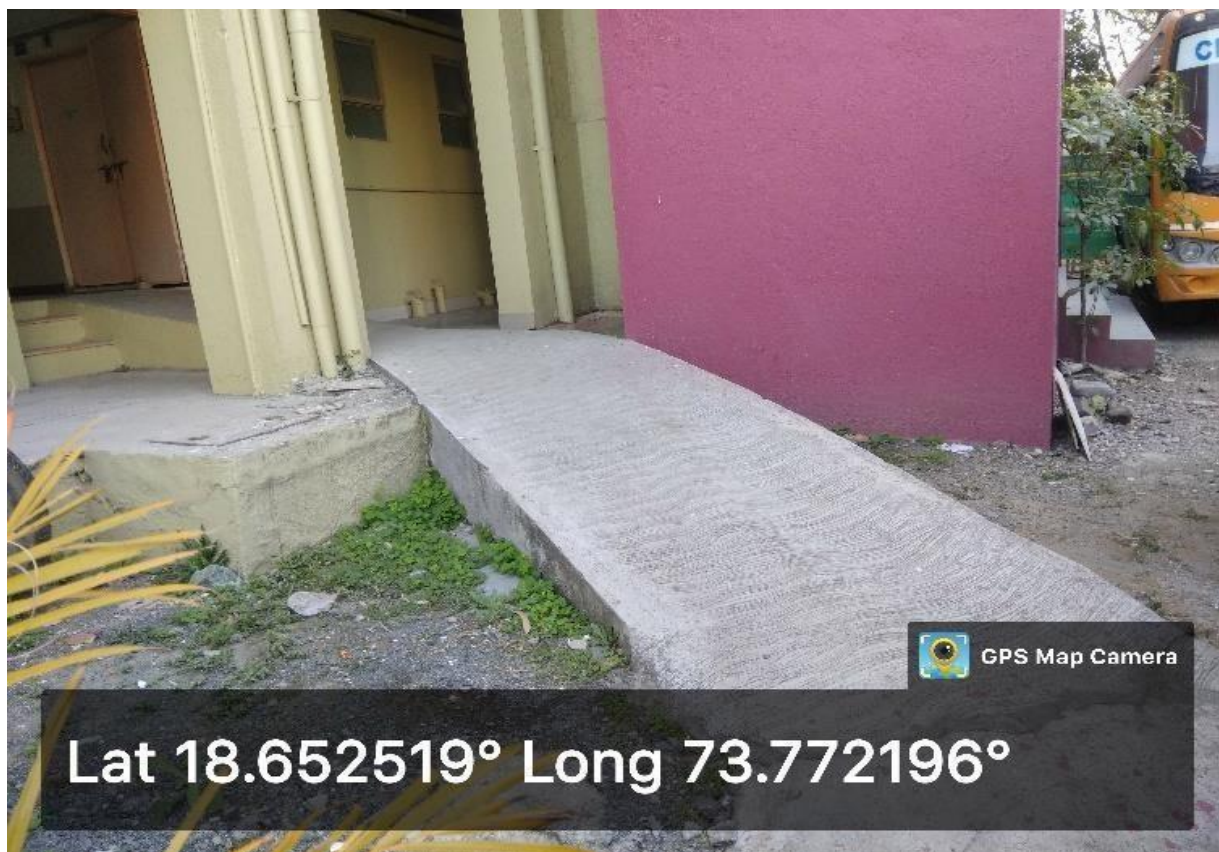
Ramp facility for handicapped
